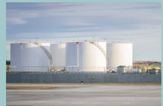
Tank to Tank
